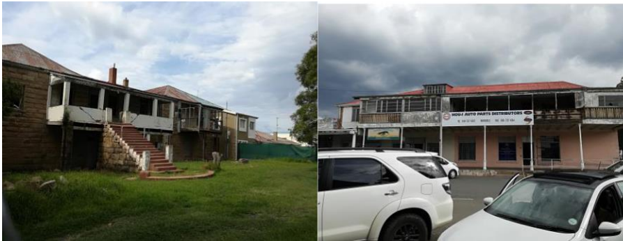
Figure 6: Examples of problem buildings around Matatiele
