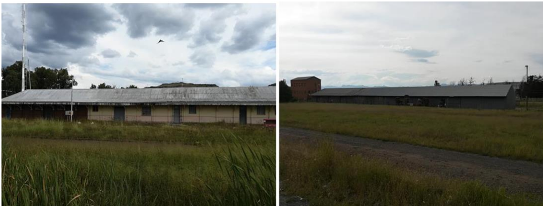
Figure 7: Dilapidated Structures around town
